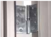
Mortise-style cam lift hinge lifts the door as it is opened to keep the bottom seal from dragging on the floor.
